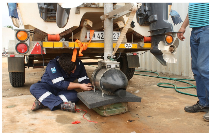
Figure 4.3: Reson SeaBat 8101 Head being mounted on pole
